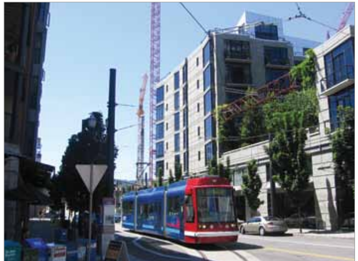
New housing under construction along streetcar route in Portland.
